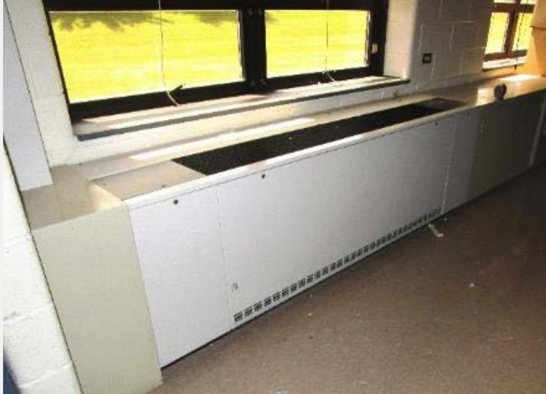
Elementary – RM 129 – UV Install/Cabinetry
